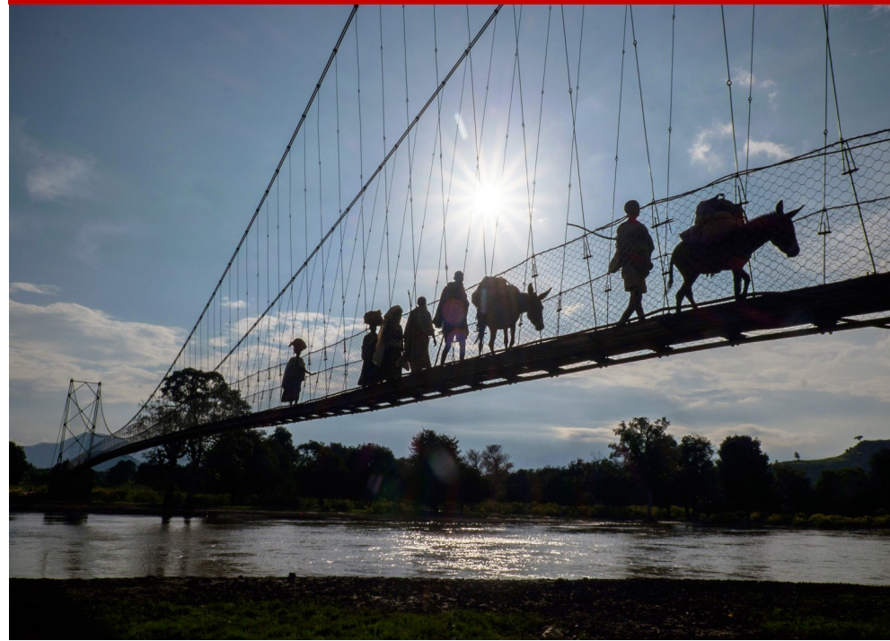
Tanquaber Bridge, located in Bahirdar Zura District
